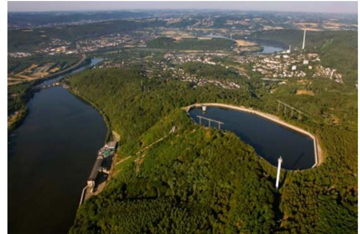
Pumped storage enables energy to be shifted from low demand times to high demand times (i.e. pump water up when the demand and price is low, generate when the demand is high and help keep prices lower)
